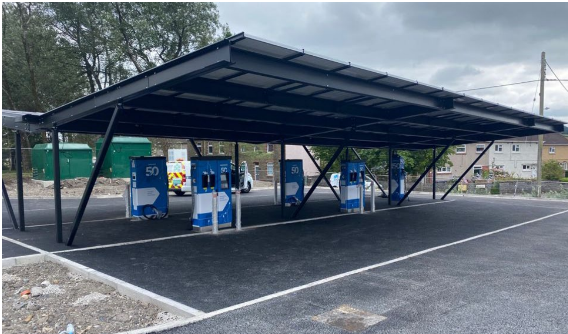
Figure 16 - Cross Hands EV Charging Hub (in construction)
